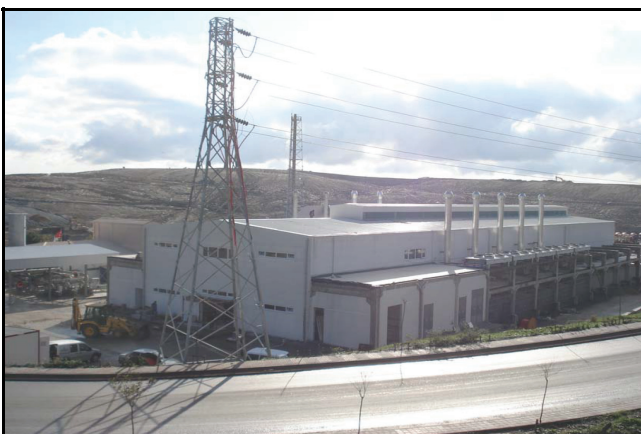
Figure 7. The plant building in the Odayeri site.
